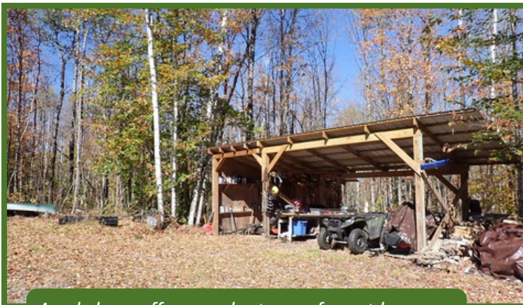
A pole barn offers ample storage for outdoor gear.
